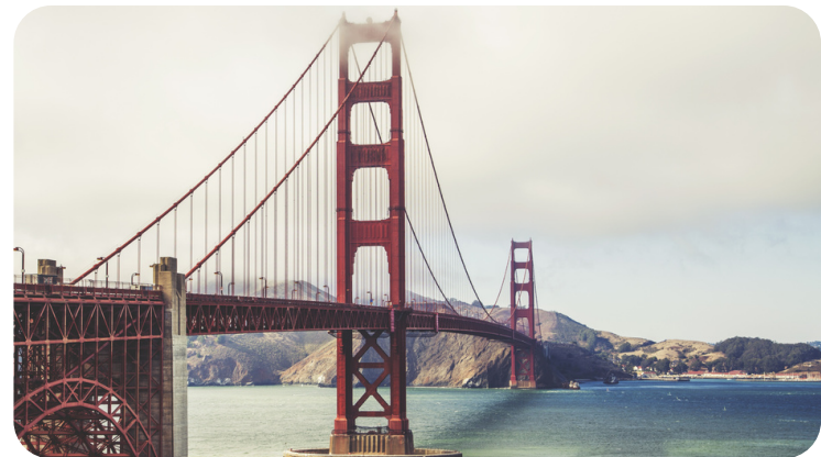
Golden Gate Bridge
